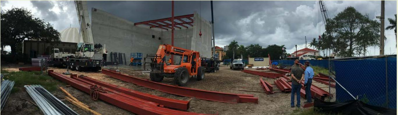
**Going Up:** The expansion – the section with the **North Education Center** and **MBU** – is about 1/3 complete. We've recently installed the structure's steel trusses and poured the rooftop concrete pad that will house its HVAC system.
